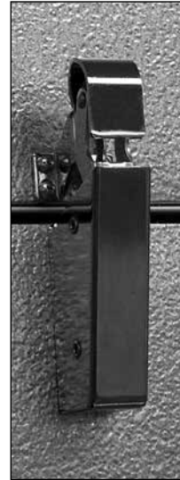
Spring actuated door closer
